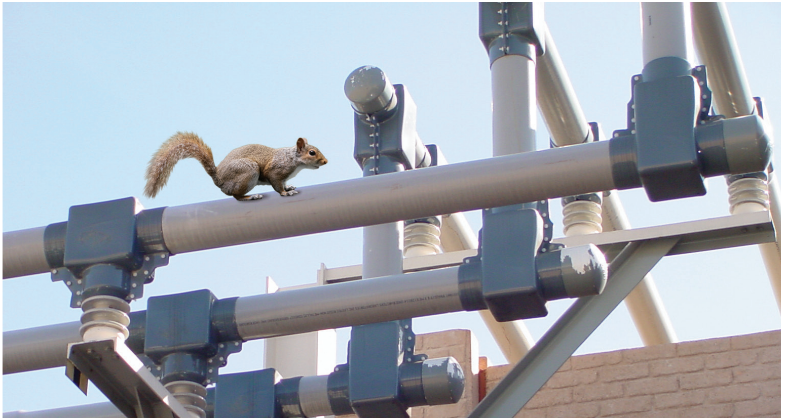
Insulboot installation in New Jersey
